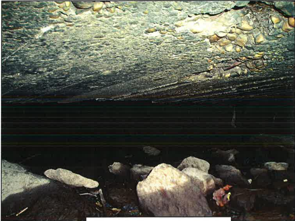
#10. Under the Downstream Slab
