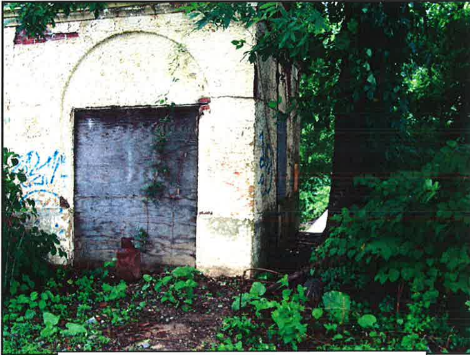
#1. Gatehouse (Filter House) on the Embankment Dam
