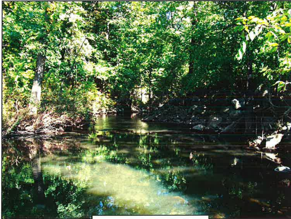
#6. Downstream of Dam
