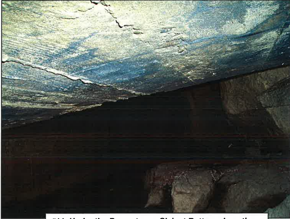
#11. Under the Downstream Slab at Buttress Location with Bedrock in Place
