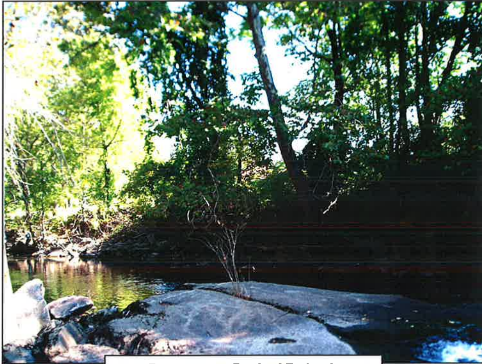
#13. Downstream Bank of Embankment
