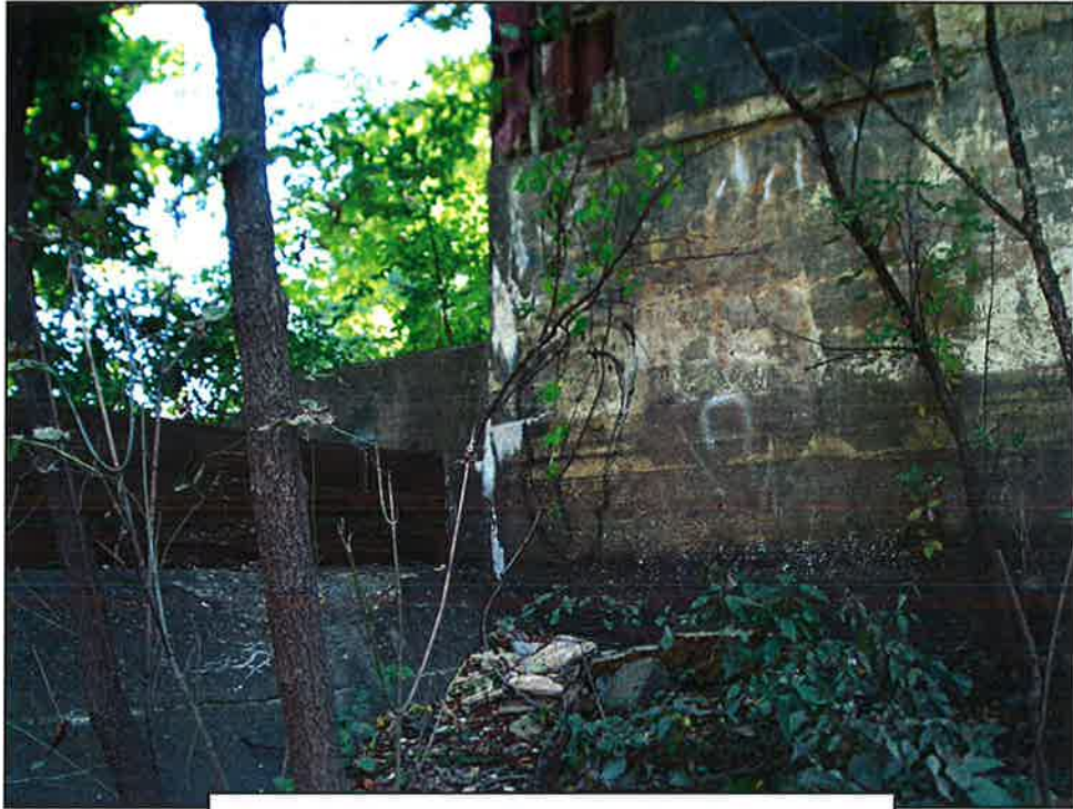
#7. Gatehouse (Filter House) and Dam Joint
